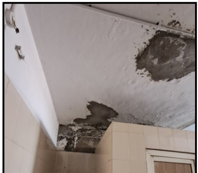
Dampness & Seepage in G.Washroom at Ground Floor
