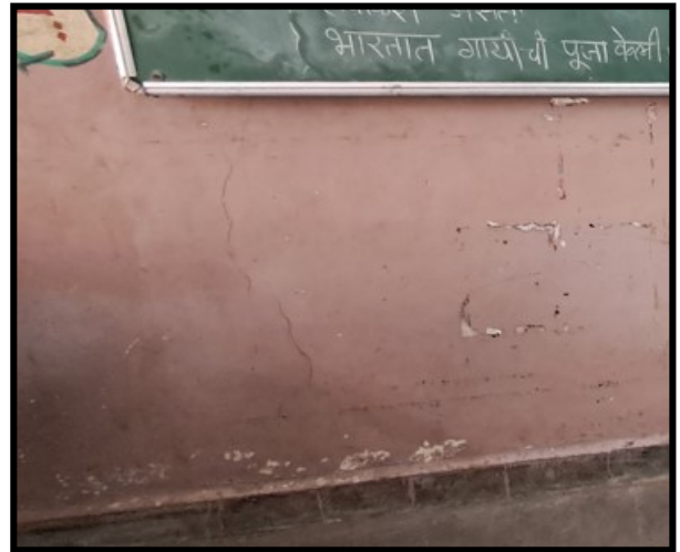
Vertical Crack in wall in Classroom 5
