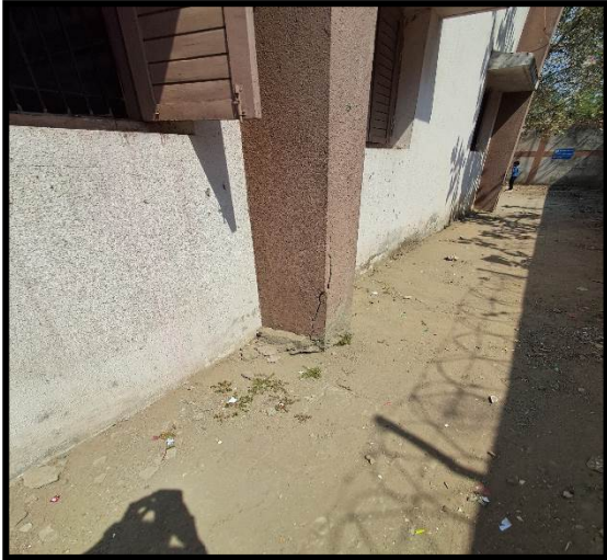
Vertical crack in Column C2 at ground floor floor
