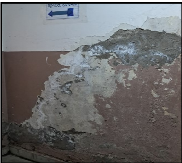
Dampness & Seepage in parab at Ground Floor
