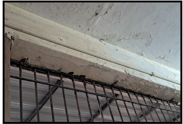
Flexural Crack in Beam 61 at Ground Floor
