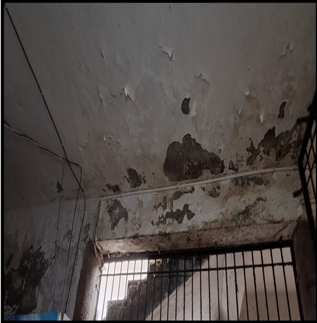
Dampness & Seepage in parab at Ground Floor
