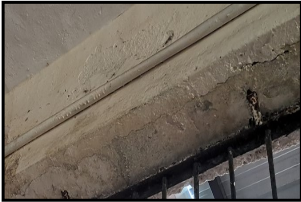
Flexural Crack in Beam 60 at Ground Floor
