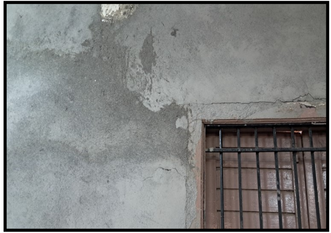
Crack Cracks in wall in Classroom 1 Ground Floor
