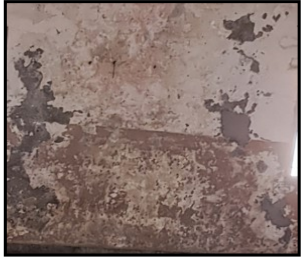
Spalling of concrete in classroom 7 Ground Floor
