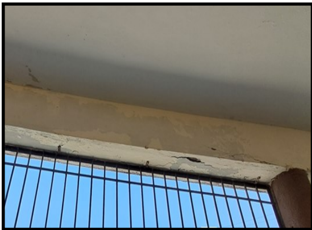
Flexural Crack in Beam 19 at First Floor
