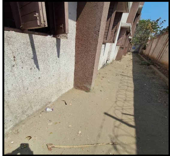
Vertical crack in Column C4 at ground
