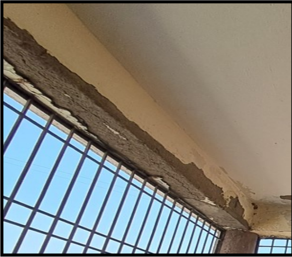
Spelling of concrete at Beam 18 First Floor
