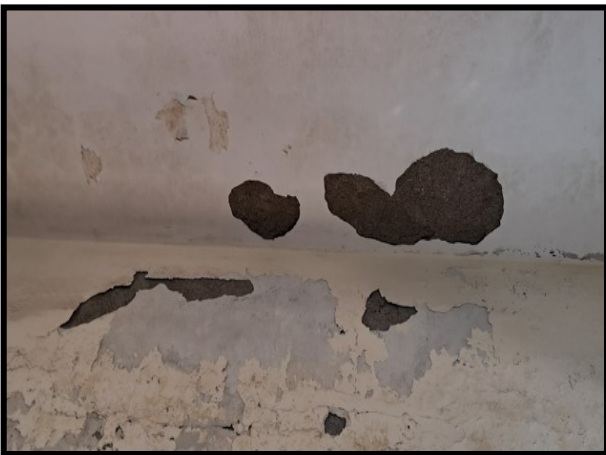
Spalling of concrete in Classroom 3 First Floor
