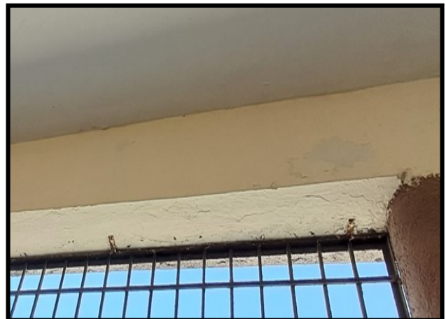
Flexural Crack in Beam 22 at First Floor
