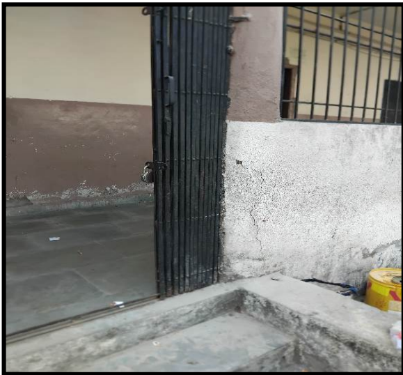
Vertical crack in Column C21 at ground floor
