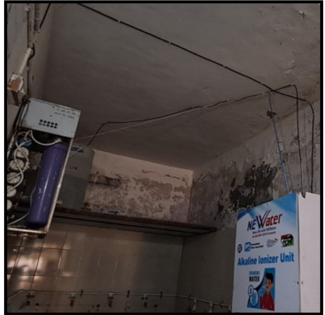
Dampness & Seepage in parab at Ground Floor
