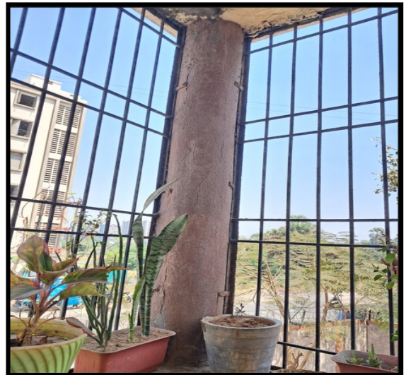
Vertical crack in Column C18 at first floor
