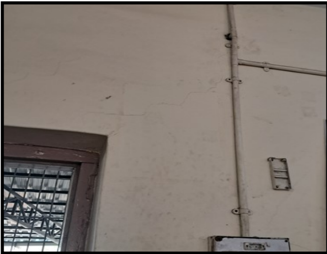
Diagonal Crack in wall in Classroom 2 Ground Floor
