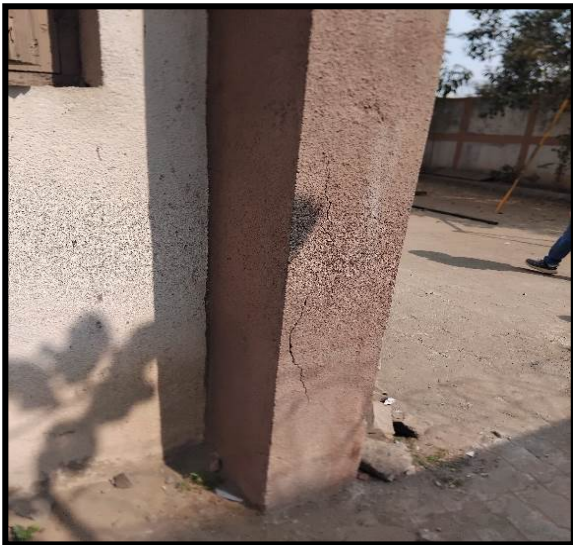
Vertical crack in Column C2 at ground floor floor
