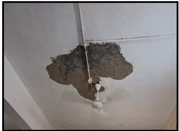
Spalling of concrete in Classroom 5 First Floor
