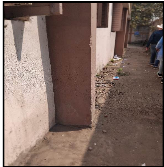
Vertical crack in Column C4 at ground
